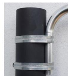
**TIP:** The Freeway can be surface mounted onto a 75mm or 100mm square post (fence posts). Alternatively, they can be mounted to metal fence supports (Metposts) using 2 x large jubilee clips. Posts are best concreted 300-400mm into the ground.
